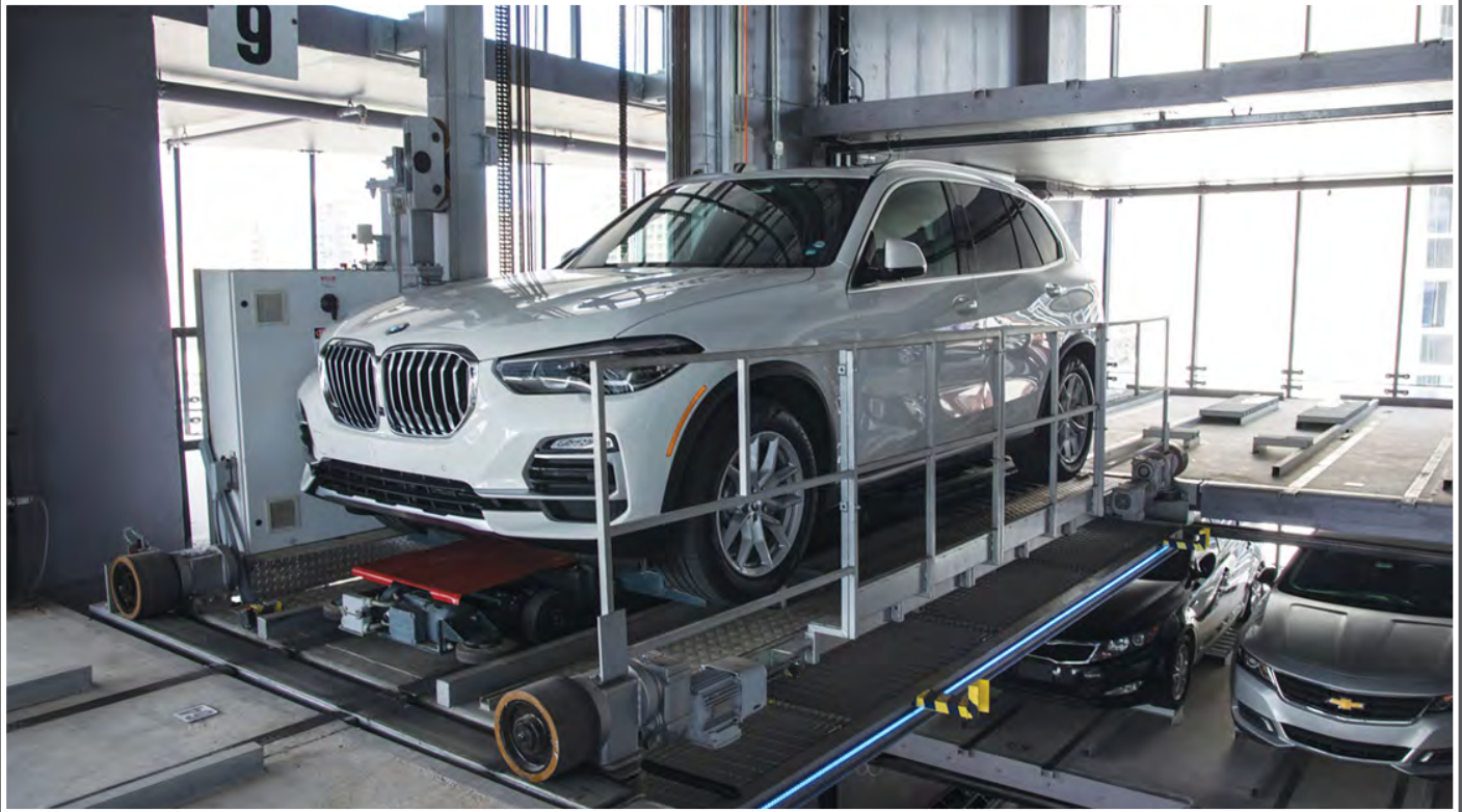
FIXED RAIL ROBOTIC SHUTTLE SYSTEM FOR AUTOMATED STORAGE AND RETRIEVAL
