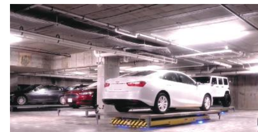
STORAGE: Vehicle is automatically parked by AGV
