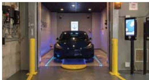
RETRIEVAL: Vehicle is presented to Loading Zone when requested
