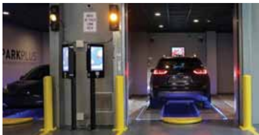
ENTRY: User parks and exits vehicle in Loading Zone
