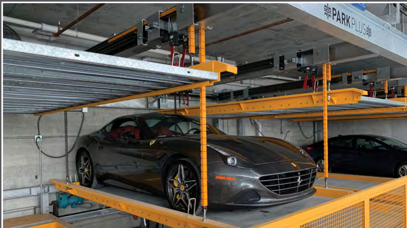
INDEPENDENT HYBRID PUZZLE STACKING SYSTEM FOR SELF-PARKING
