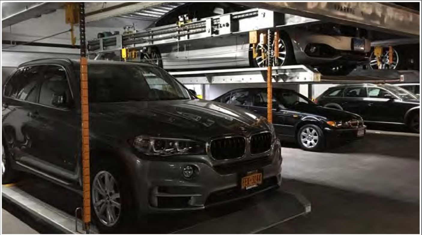
2-HIGH SUSPENDED SYSTEM WITH BUILDING INTEGRATION FOR COLUMN-FREE STACKING
